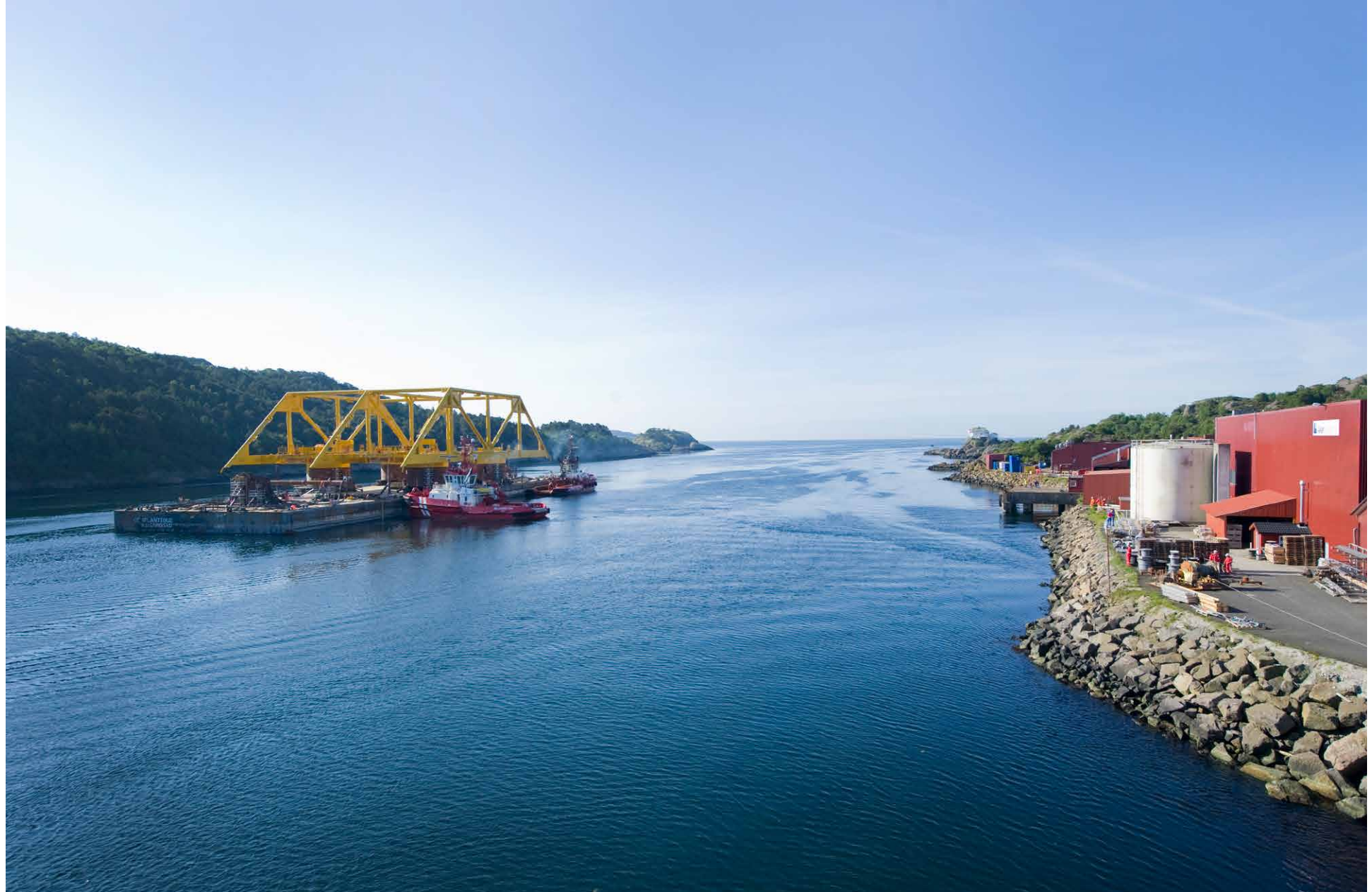
In June 2013, Aker Solutions delivered the steel frame for the world's first subsea gas compression facility to be installed at the Statoil-operated Åsgard field.
